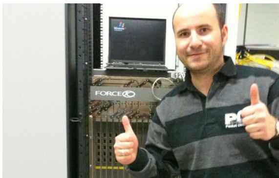
DE-CIX' Daniel Melzer after successful implementation of the first Force10 Exascale switch, internal ID „switch21“
